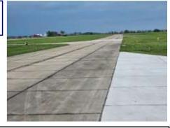
When concrete was tested, it fell below the acceptable percentage of strength to be repaired and requires replacement, causing review and reapproval of the project by FAA. Project delayed from 2024 to 2025.
